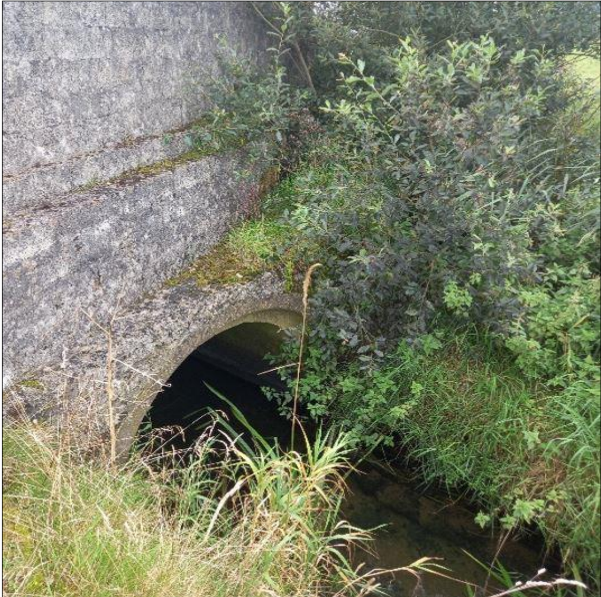
Plate 10.4: Watercourse crossing, looking north west
